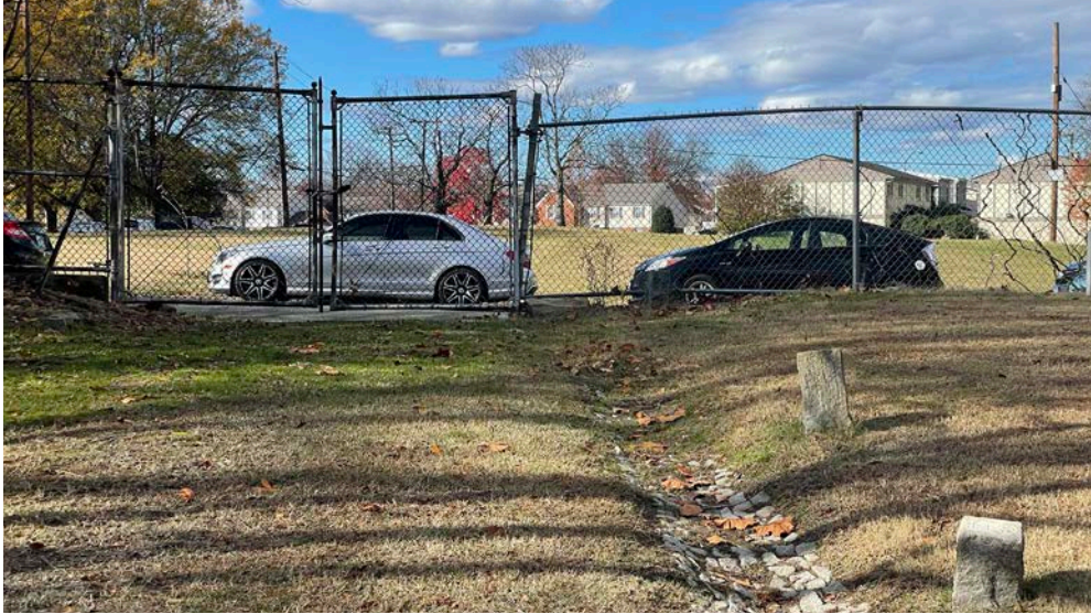
Existing gate and fence to be replaced on Dobson Street
