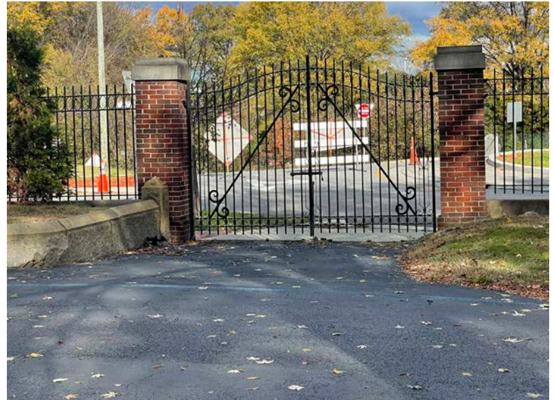
Gate and fence to be installed
