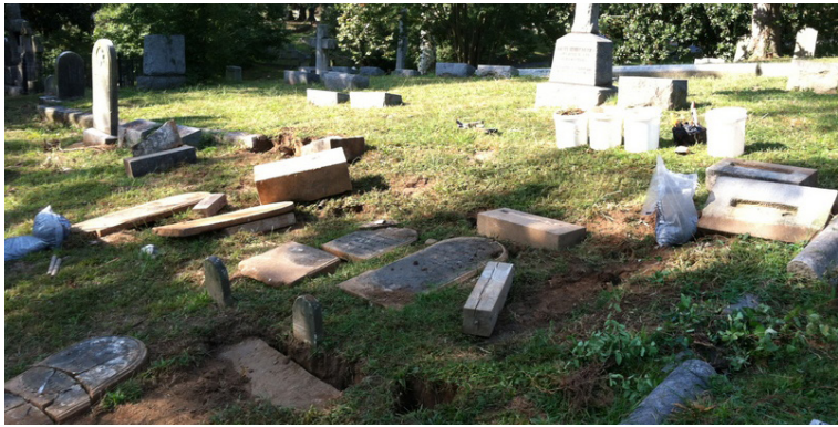
The condition of the Norton plot before repair and restoration earlier this year. Topped and broken tablets, dislocated bases, a mess!
